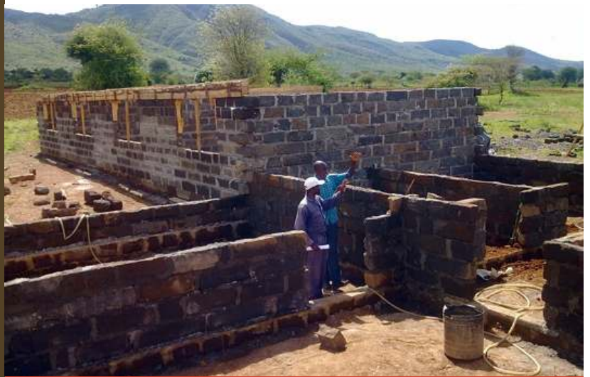
Walls of new high school being built at EBCCK
